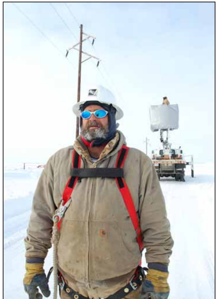
Bruce Christensen and his fellow NIPCO crewmen braved snow, ice and cold temperatures to turn the lights back on in South Dakota. (Photo courtesy of East River Electric Power Cooperative)
