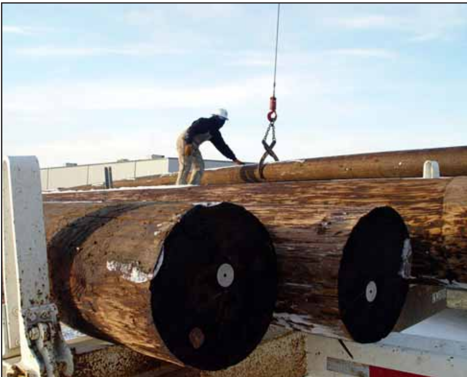
Jim Marco helps load wood poles before he and four other NIPCO crewmen left for 10 days of work helping restore the storm-damaged East River Electric Power Cooperative system.
