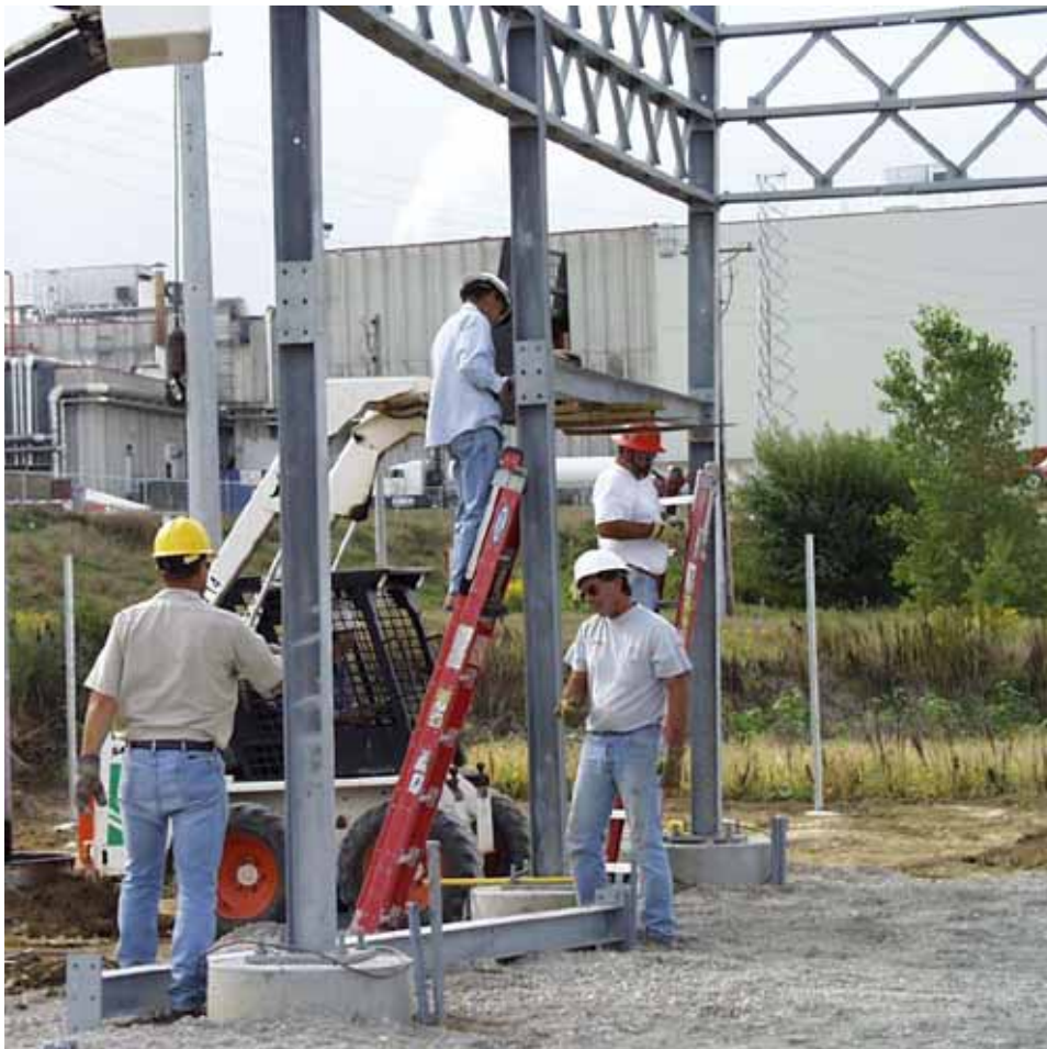
The price of structural steel has increased during the past year. Here NIPCO crews assemble steel at the new Southern Substation in Oakland. (Photo courtesy of Mary Johnson, Nishnabotna Valley REC)
